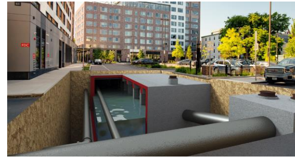
Screenshot from https://www.kleinfelder.com/project/pl6-stormwater-storage-tank-tunnel/
