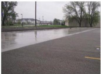
Figure 3-4 Permeable concrete adjacent to traditional concrete during a rainfall, Ames, IA Source: John Kevern
